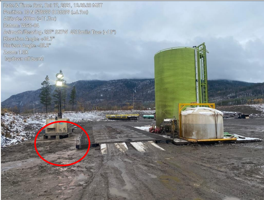
Photo 41. Overview of wash station. Red circle indicates location where wash station is discharging hydrocarbon laden water to the environment.
