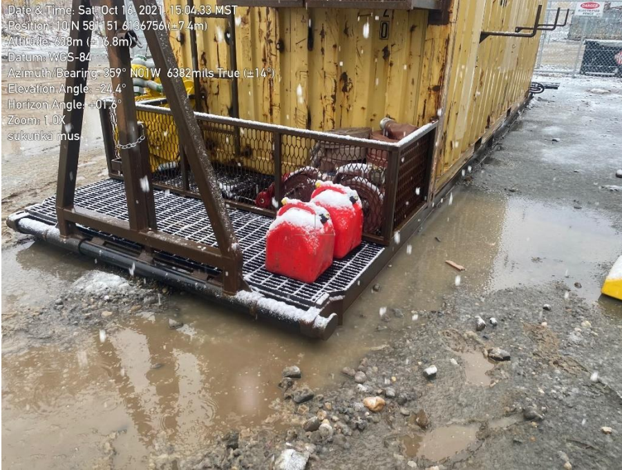
Photo 26. Jerry cans without secondary containment.
