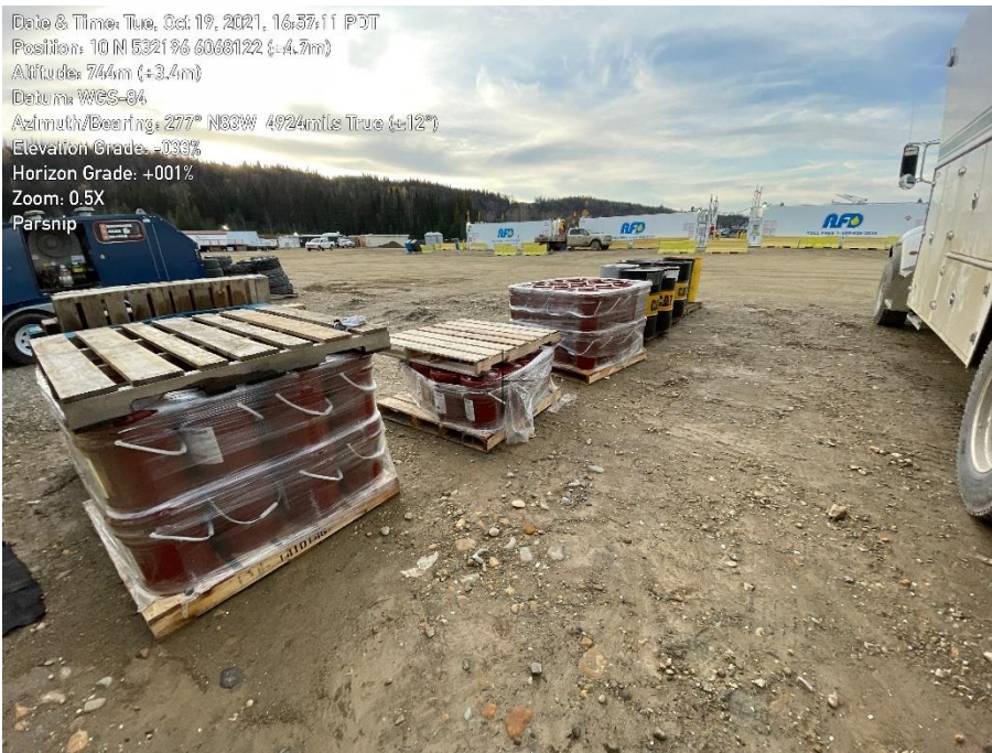
Photo 27. Bulk chemical liquids stored without secondary containment- Parsnip MUS.
