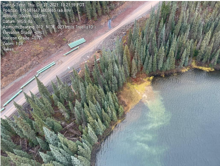
Photo 6. Example of Project inputs into lakes between KP586+600 to 587+500 as seen from air.
