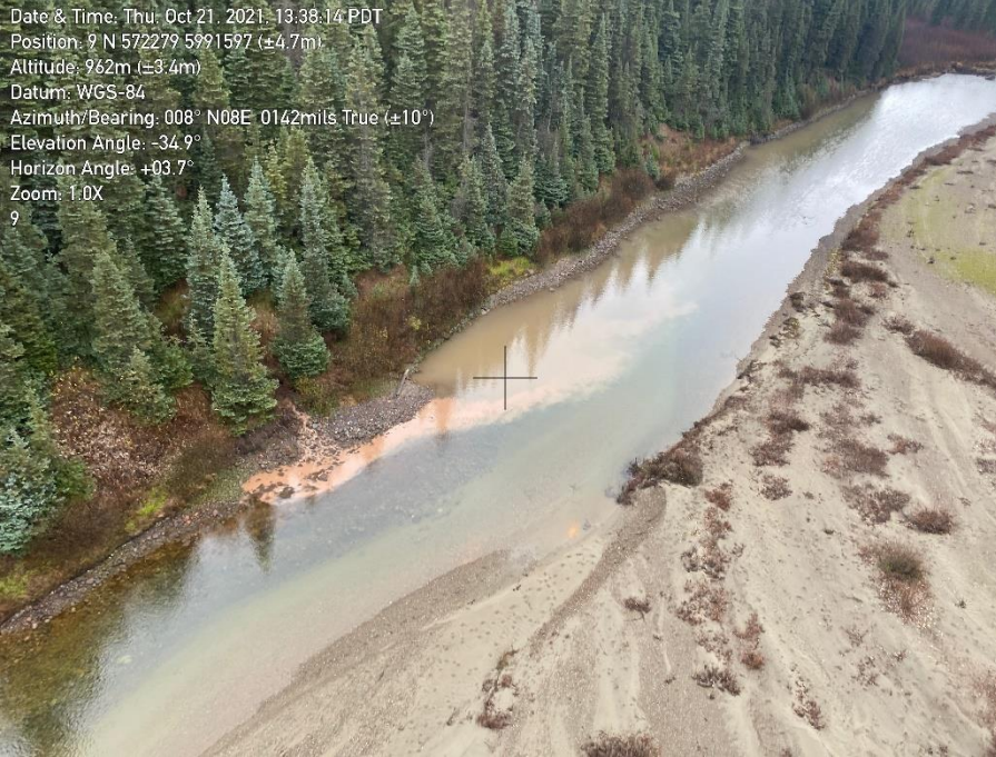
Photo 7. Example of Project inputs into the Clore River as seen from air.
