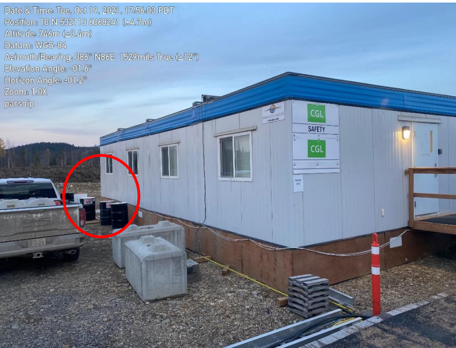
Photo 35. Overview of storage area, near site offices. Note barrels without secondary containment in place (Requirement 4, above).
